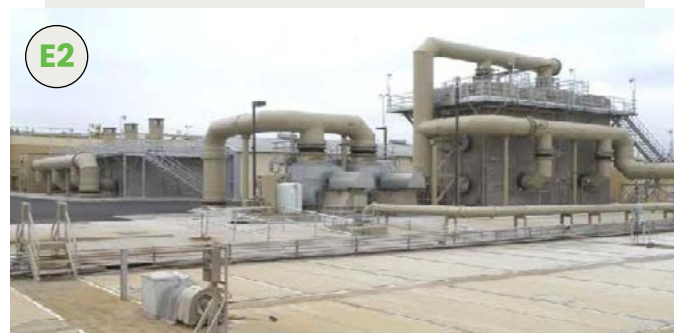
The four odor control cells retrofitted with Cell-Max™ demonstrated substantial improvements in H 2 S treatment effectiveness
