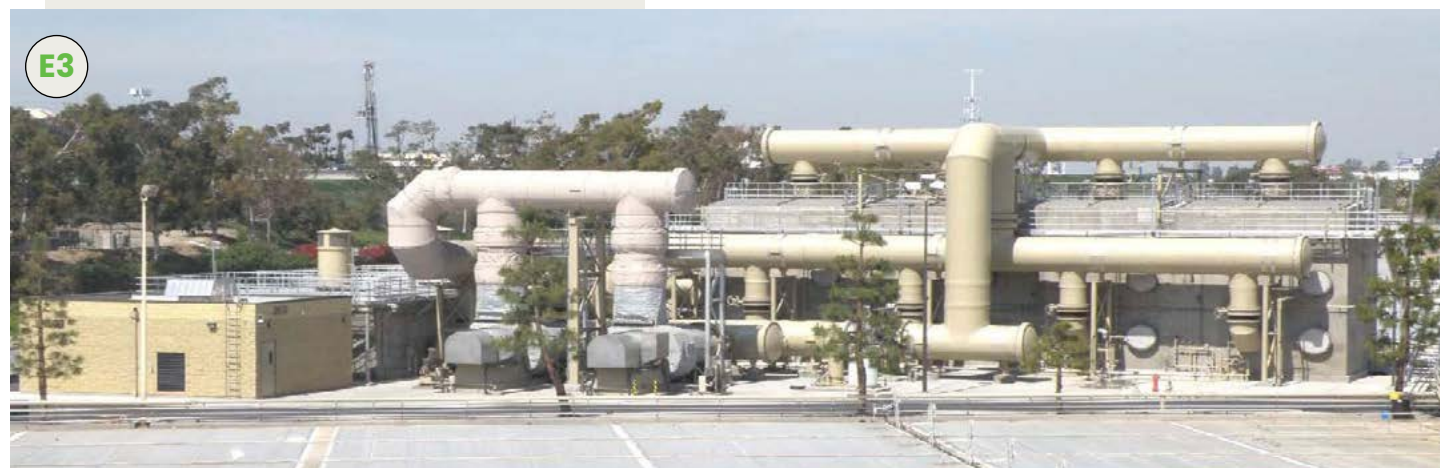
The four odor control cells retrofitted with Cell-Max™ demonstrated substantial improvements in H 2 S treatment effectiveness
